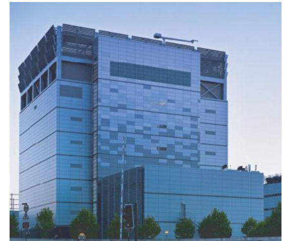
Telehouse Docklands data centre
